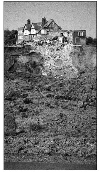
Figure 5. Wreckage of the Holbeck Hall Hotel is strewn down the headscar of the landslide that destroyed it at Scarborough in 1993.
