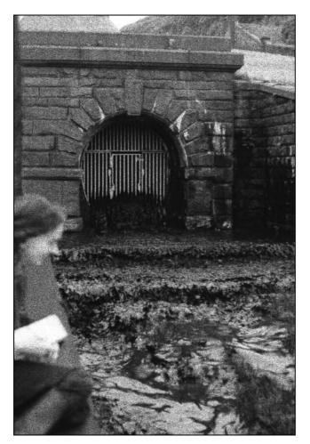
Figure 6. Sediment-rich water released on opening the bottom scour valve at Blakeley Reservoir, Yorkshire
